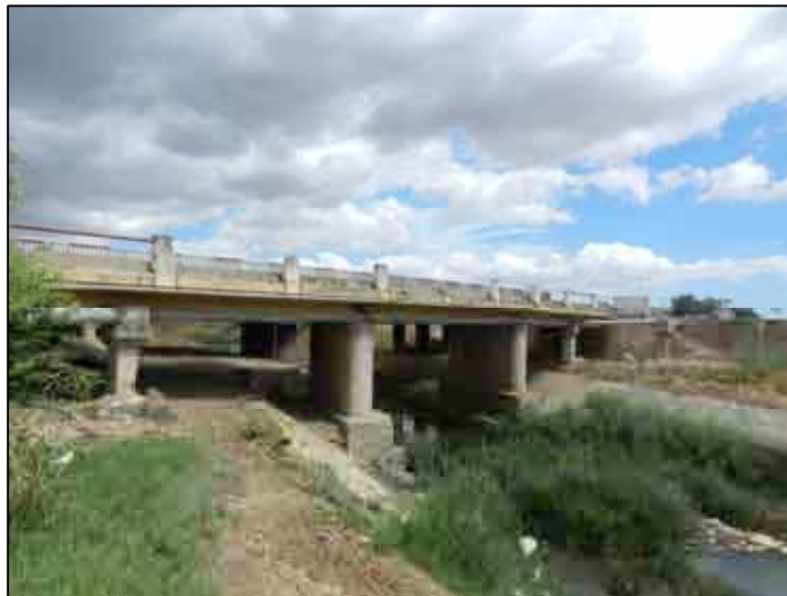
Figure 6.3-12 Current Status of GP7 Old Bridge on Chafrou(Aug., 2012)
