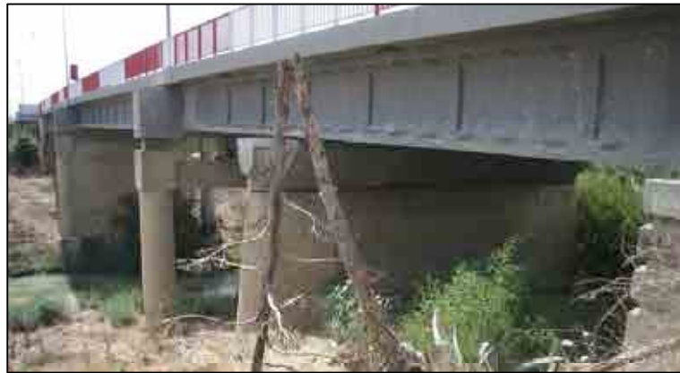
Figure 6.3-10 Current Status of Jedeida Bridge on GP7 (Aug., 2012)
