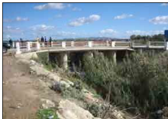
Figure 6.3-14 Current Status of El H'Bibia Bridge (Aug., 2012)
