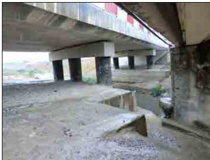
Figure 6.3-11 Current Status of GP7 Bridge on Chafrou (Aug., 2012)
