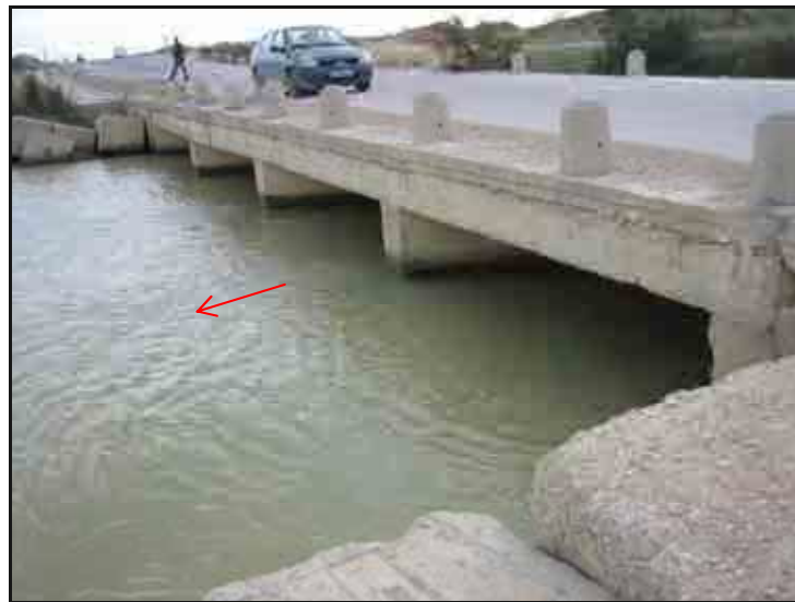
Figure 6.3-1 K. Andalous Bridge in August 2012
