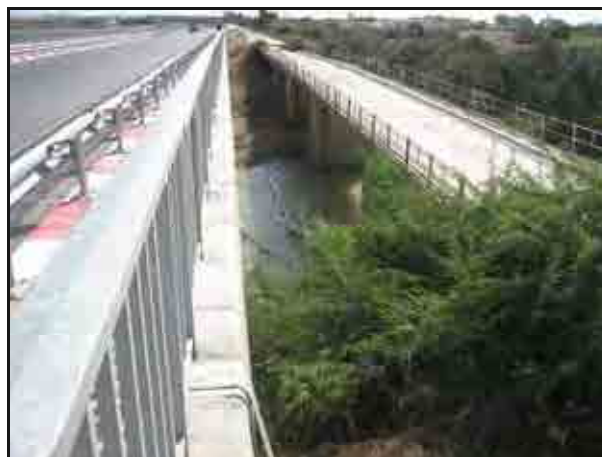
Figure 6.3-3 Tobias Old Bridge in August 2012
