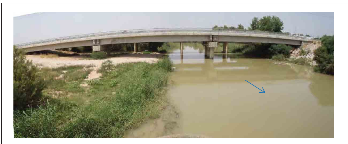
24. Tobias canal gates – immediately upstream of the bridge (2012.08)
