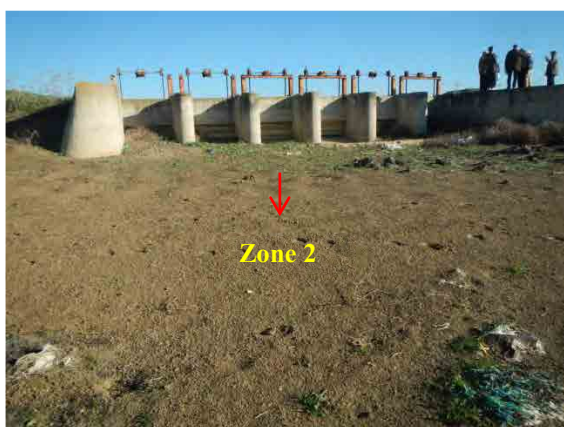
Figure 3-23 Overflow Weir (Zone 3 to Zone 2) with Gate
