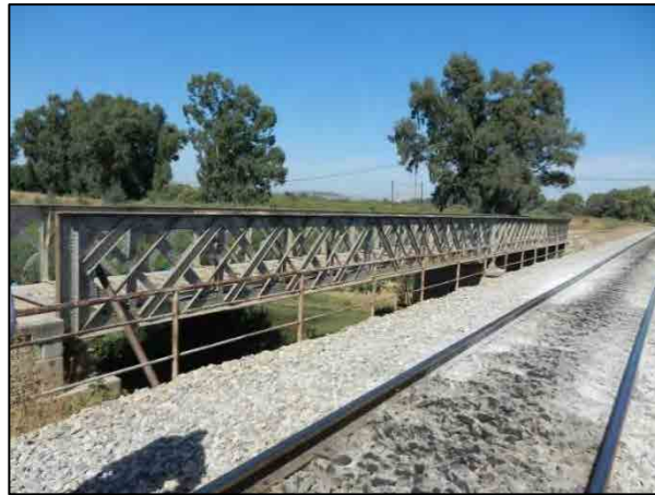
図 6.3-7 Jedaida Railway Old Bridge 橋の現況 (2012.8)
