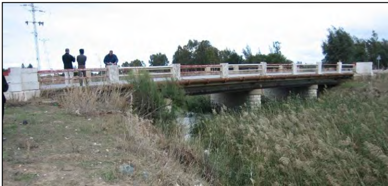
図 6.3-20 GP8 Bridge and Road Over Mabtouh 橋の現況 (2012.8)
