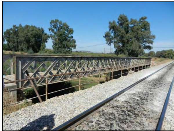
図 6.3-7 Jedeida Railway Old Bridge 橋の現況 (2012.8)
