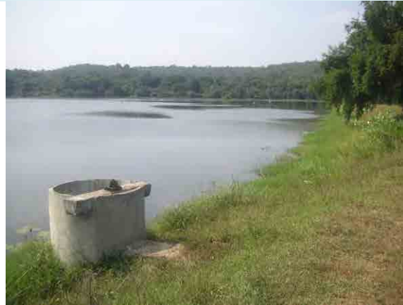
Irrigation Tank (Trincomalee)
