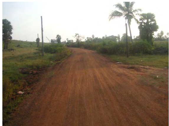
Rehabilitated Rural Road (Manner) National and Province Road rehabilitation work is going on under several projects in dry zone with ADB and other fund
