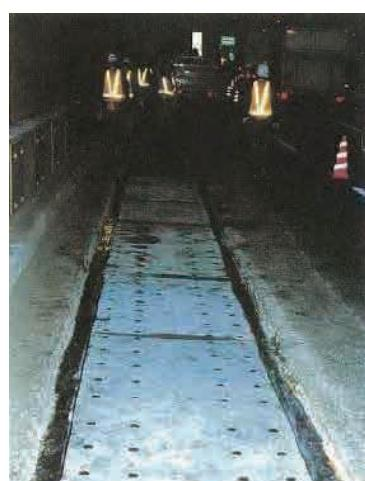
**Photo 1 Reinforcing Plate of the Steel Deck Plate**
