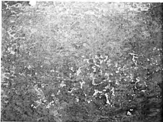
Photo-5 Corrosion roughness on steel deck plate
