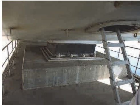
Photo 6.1.3 Entrance Manhole of Steel Deck Girder
