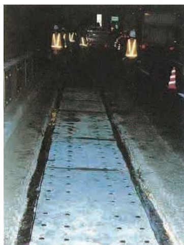
Photo 1 Reinforcing Plate of the Steel Deck Plate
