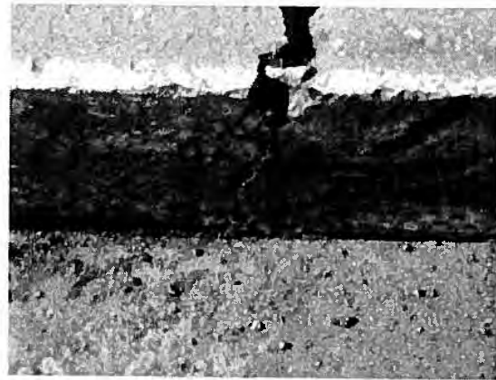
Photo-2 Crack with 10mm width reaches into Binder Layer
