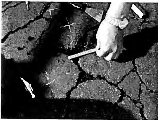
Photo-1 Crack Condition
