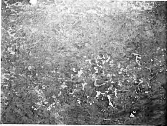
Photo-5 Corrosion roughness on steel deck plate
