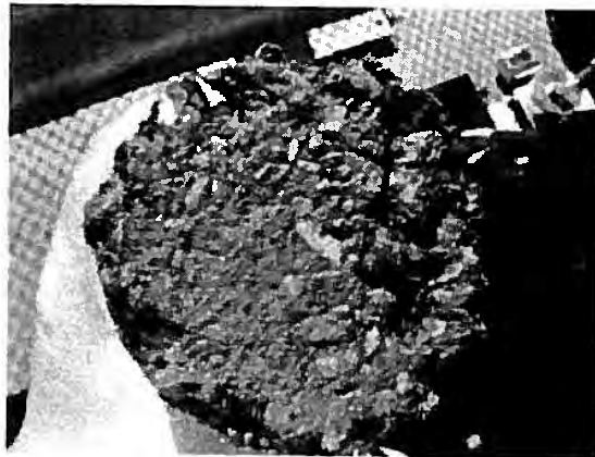
Photo-4 Failure of Bonding Layer
