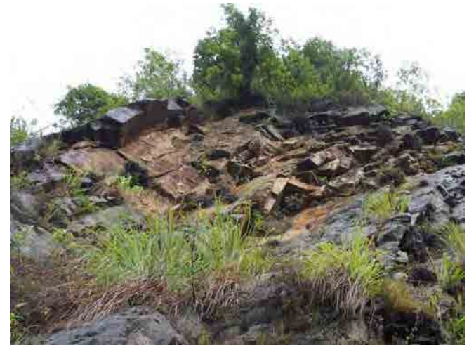
Condition of the lower slope. From the shoulder of the road, very steep lower slope descends downward.
