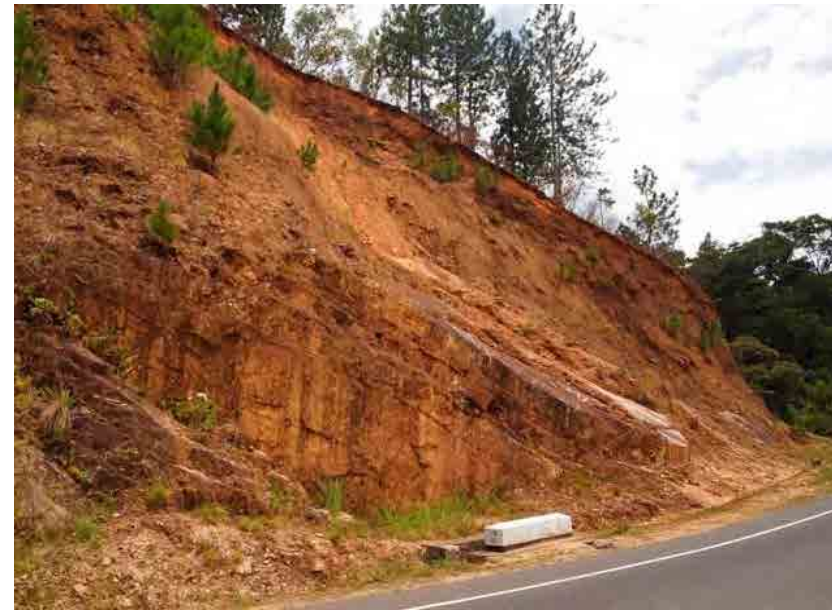
Condition of slope, basement rock of dip slope structure
