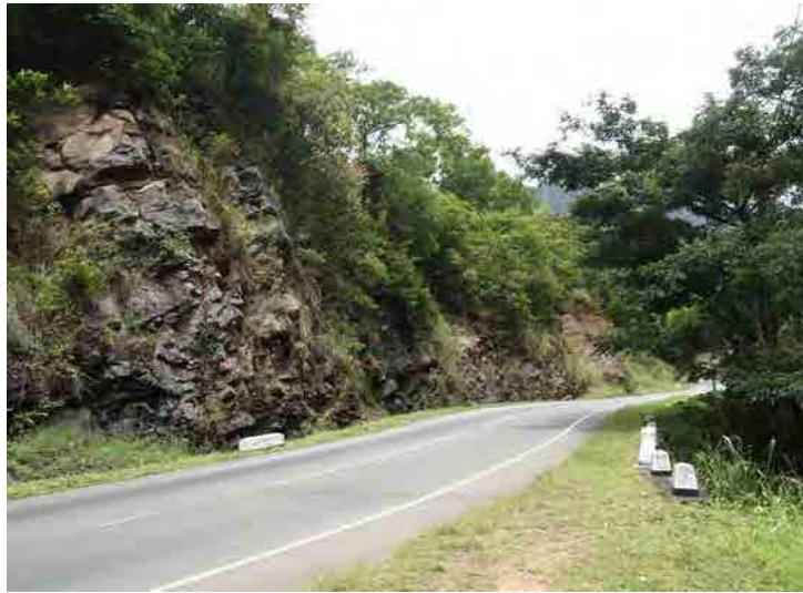
Full view of the slope at the ending side
