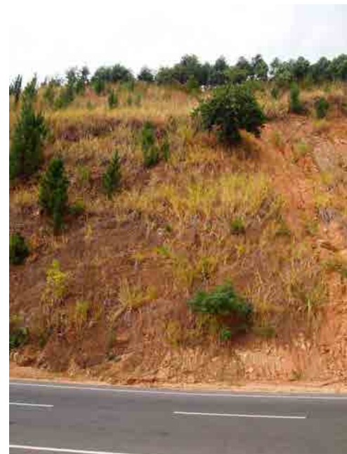
Condition of slope, the slope on the start side is a slope of a steady sedimentary rock
