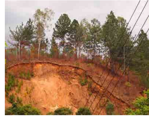
Situation of slope head
