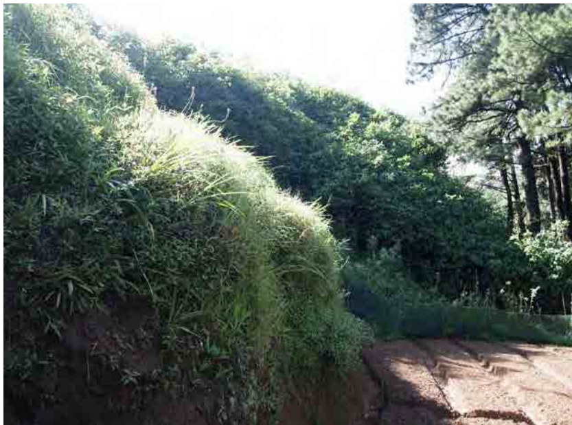
Condition of slope, state of road lower slope
