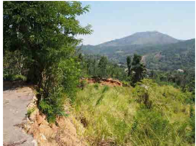
Escarpment of a divided landslide.
