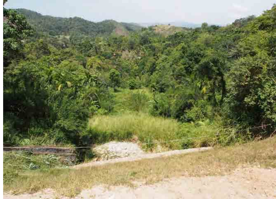
Situation under slope
