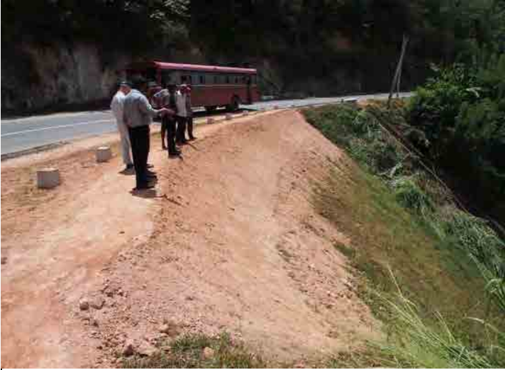
Full view of the slope at the beginning side
