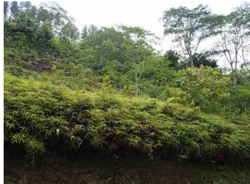
Adjoining old collapse ground
