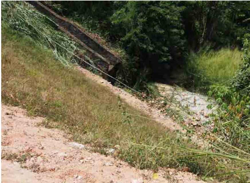
Condition of slope
