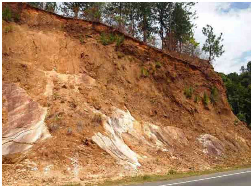
Condition of slope, a loose sedimentary soil is recorded on the base rock.
