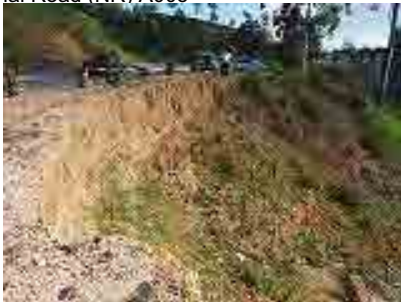
ii) Head scarp of a divided landslide just beside the main road at NR A016
