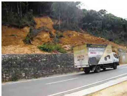
Figure 3-8: Gabion Walls (A-5 Road, km 192)
