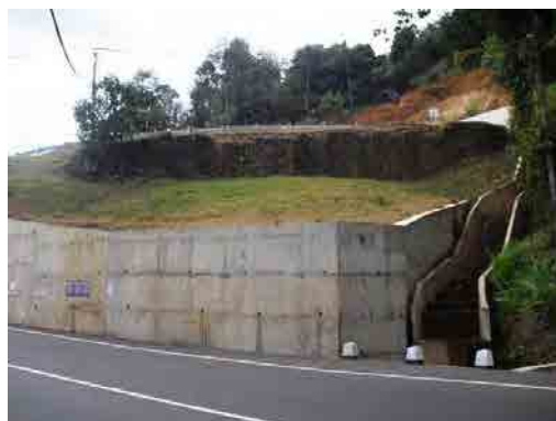
Figure 3-7: RC Retaining Wall at A-26 Road (Kandy)
