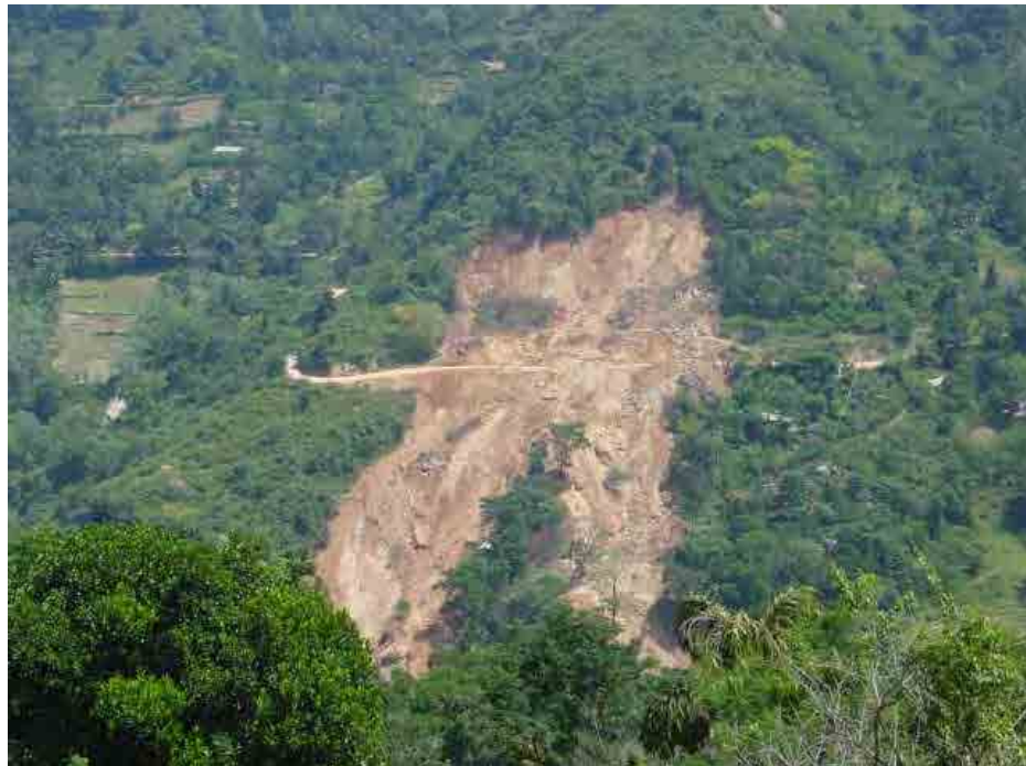
Figure 2-21: Landslide at Walapane(photo by Mr.Tsukamoto)
