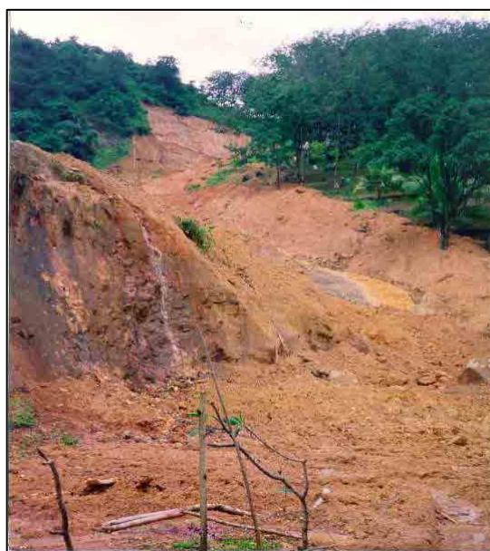
Figure 2-19: Earthflow at Helauda (photo by NBRO)
