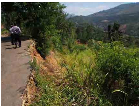
Figure 4-6: Condition of the landslide of A005-135
