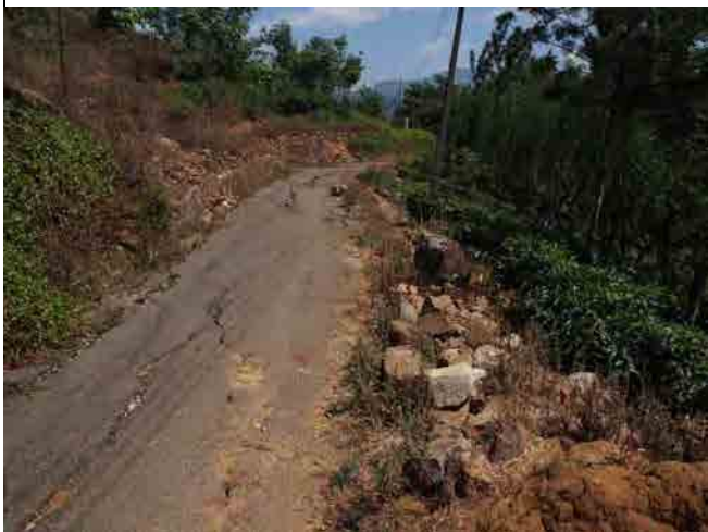
Cracks at the middle of landslide.
