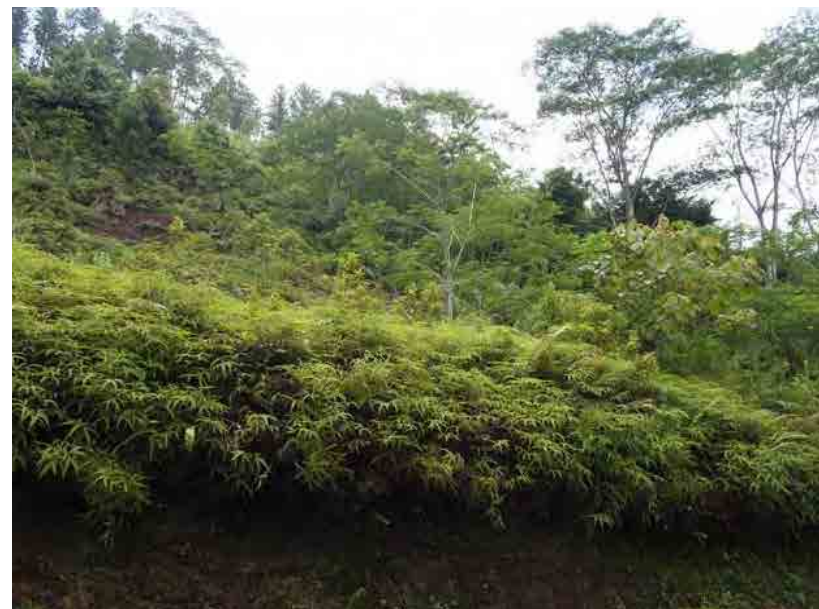
Adjoining old collapse ground
