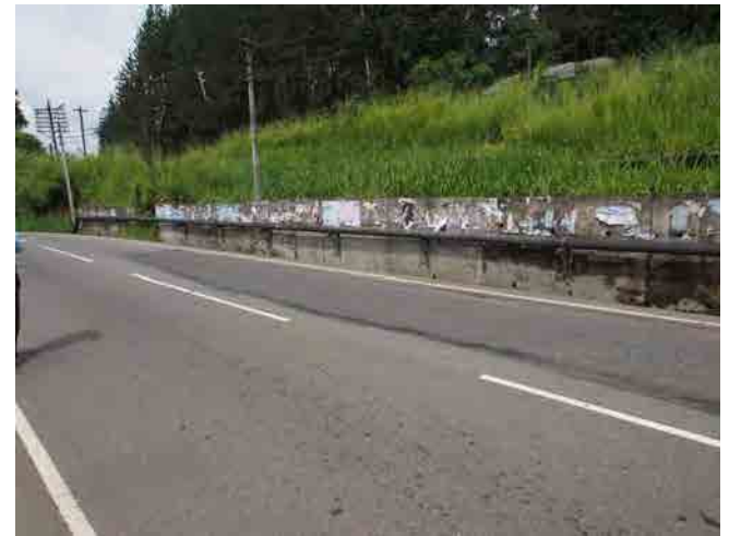
Retaining wall along the road. After the construction of this retaining wall, landslide of upper slope was said to be eased.
