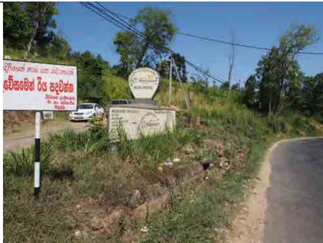
Toe of the landslide. Hospitals and houses were destroyed by the landslide movement.
