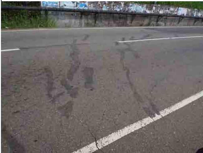
Cracks appeared on the road surface. Cracks seem to follow the shape of a head scarp under the pavement.
