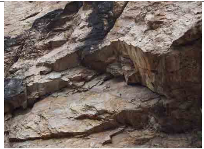
Sheeting joints notably developed parallel to the slope.
