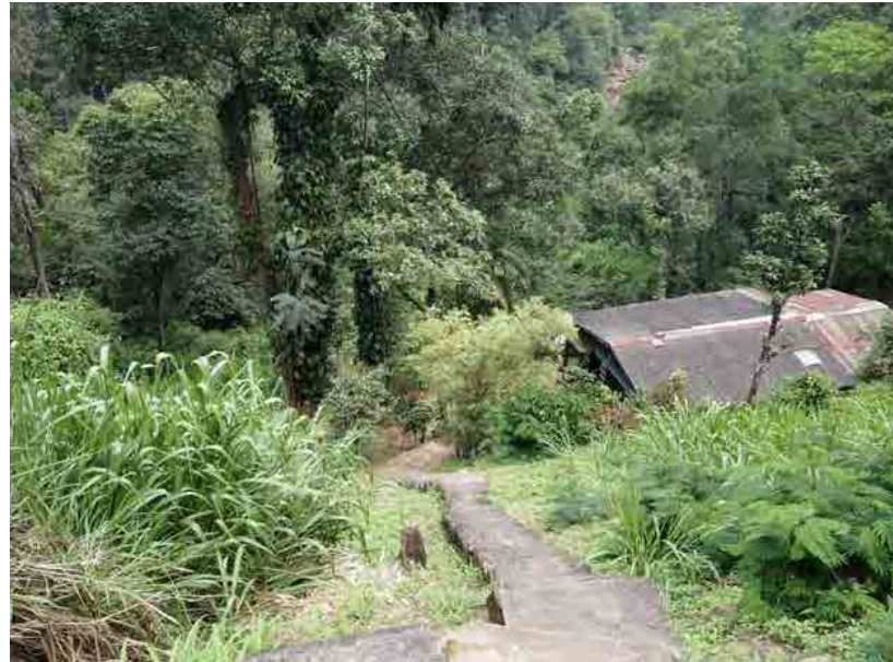
Condition of slope, house under slope
