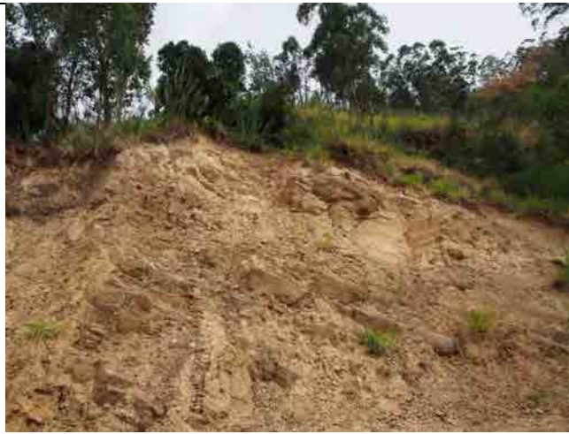
Condition of the slope. Heavily weathered condition are understood. Foliation and cracks developed densely and helped weathering proceed.
