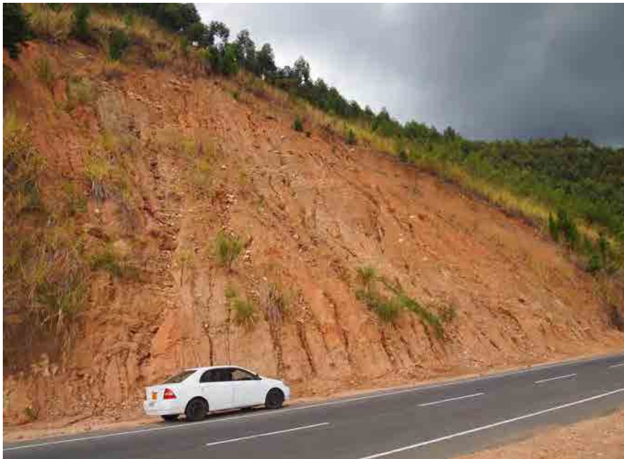
Condition of slope, many can confirm the mark of erosion
