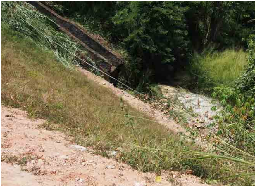
Condition of slope
