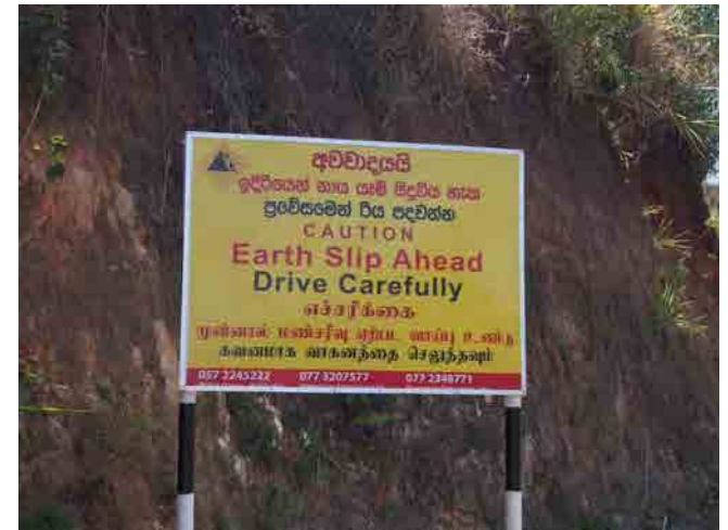
Signboard warning the landslide
