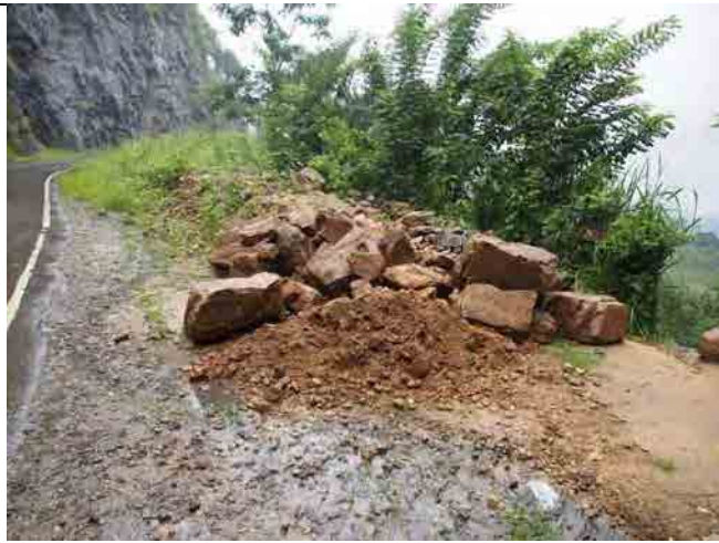
Debris cleared up to the shoulder of the road
