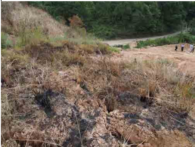
Open cracks were seen at the middle of the landslide.
