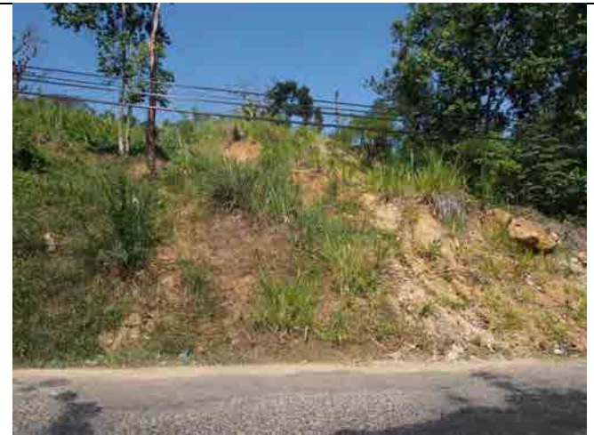
Toe of the landslide. Debris from the landslide accumulated and closed the road when the landslide was activated.
