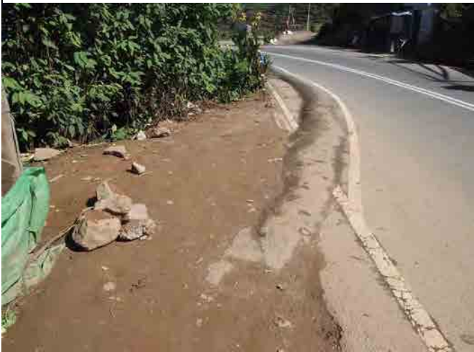
Full view of the slope from strat side
