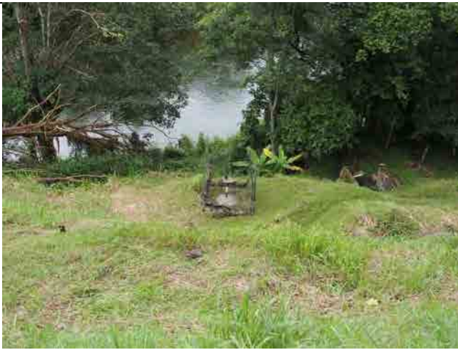
Piezometer installed at the lower part of the landslide.
