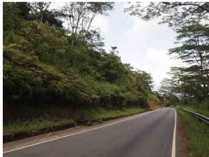
Full view of the slope from end side
