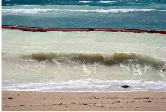
Photo 14.5.7 Separation Screen for Preventing Turbidity Diffusion
