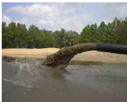
Photo 14.5.5 Direct Discharge of Sand by Pipe
