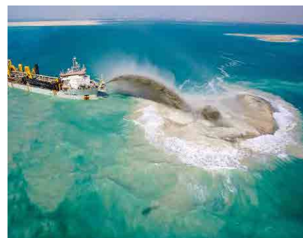
Photo 14.5.6 Direct Discharge of Sand by Ship
