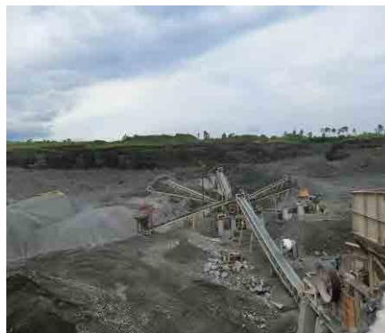
Andesite Quarry Plant
