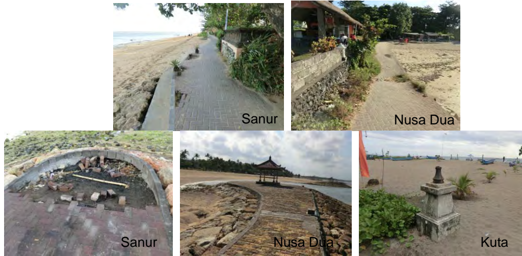
Photo 2.2.3 Damages to Public Facilities
