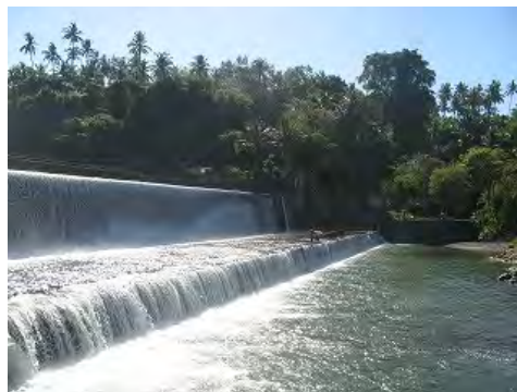
(2) Weir for Irrigation
