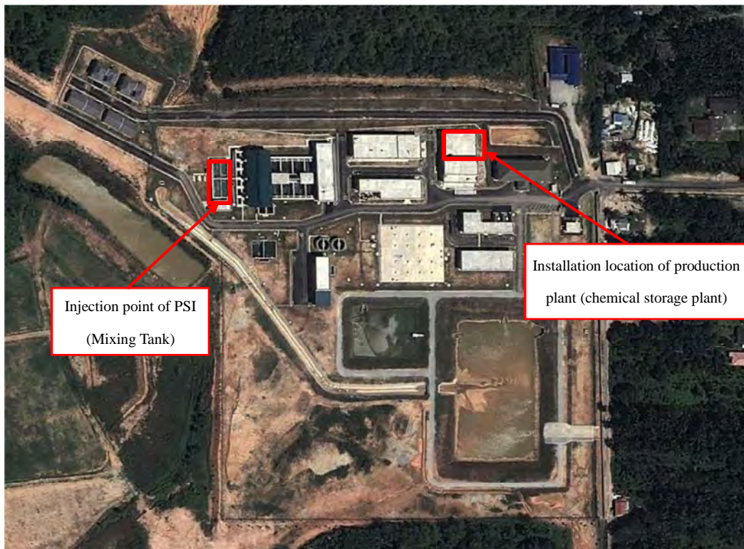
Fig. 4.3 Overview of installation location of facility (LABU water treatment plant)
