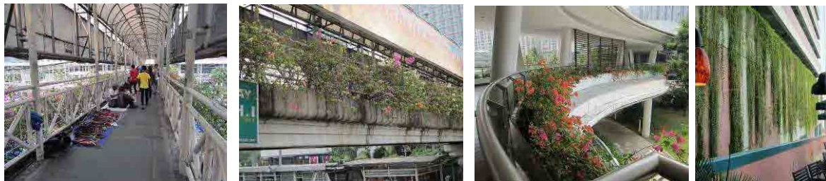
Public pedestrian bridge
