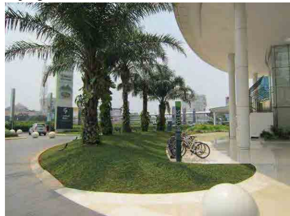
Providing depth for planting using an embankment
