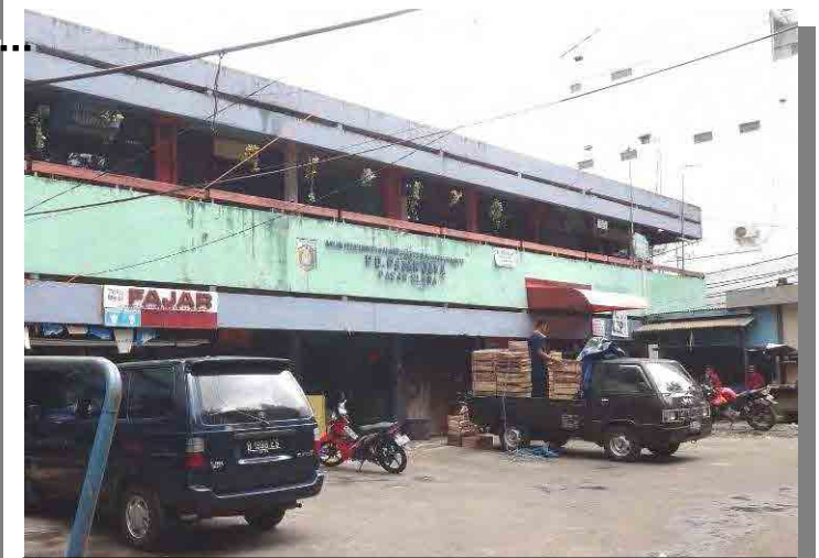
Public market PASAR BLORA standing on public space
