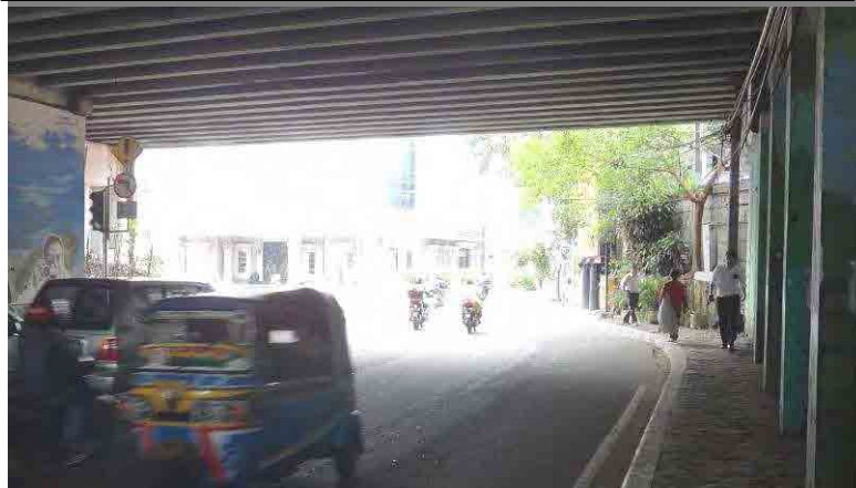
The width of the pedestrian walkway on Dukuh Atas Bridge north side tunnel is less than 2m, but still during rush hour it is used by many pedestrians
