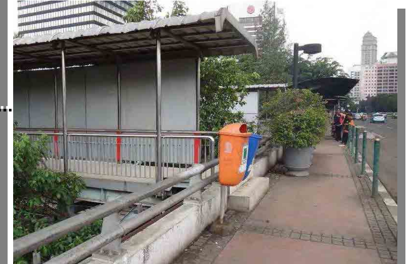
Connection between Sudirman Railway Station and Dukuh Atas Bridge
