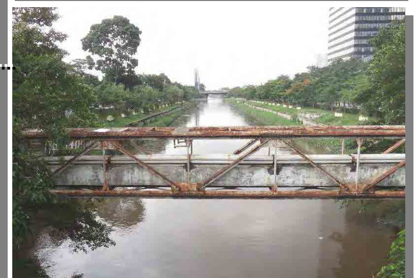
Pipe bridge crossing the river (Banjir Kanal)
