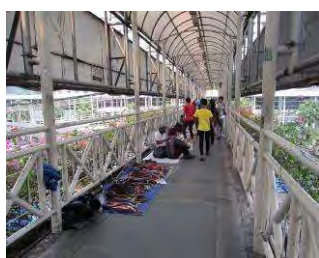
Public pedestrian bridge
