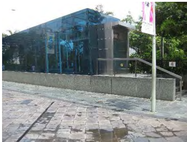
Figure. 4.3.49 Artist's depiction of flood control measures for underground connecting passageway (Singapore underground passageway entrance Source: Study Team)
