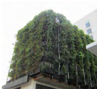
Wall surface greenery using a mesh (applied to bridge piers) (vines)
