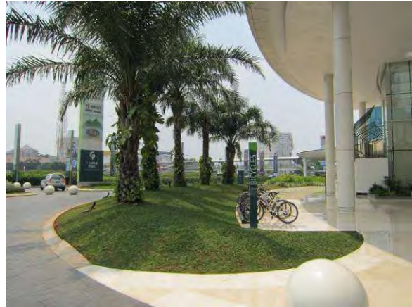
Providing depth for planting using an embankment
