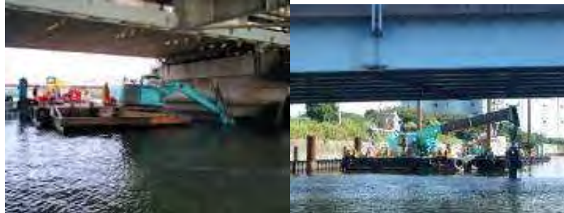
Figure-4.3.36 Dredging with a crane (left) and backhoe (right) placed on a barge
