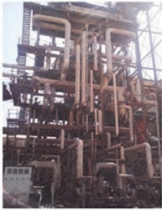
Ammonia Plant Structure
