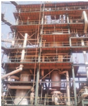
Urea Plant Structure
