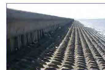
recommended dyke for erosion protection 2.500.000 USD/km
