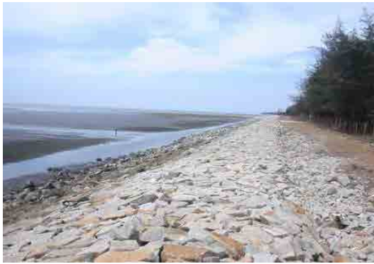
Reference for Riprap (Source: ICOE)
