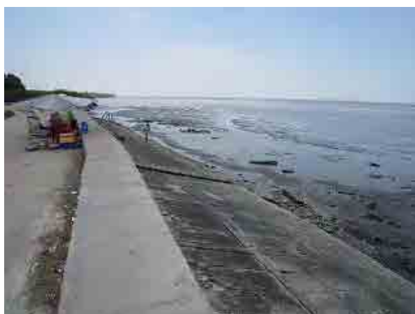
Left photo shows a typical concrete strengthened sea dyke, and the right photo shows mangrove reforestation combined with wave dissipater constructed with concrete frame packed with stones.
