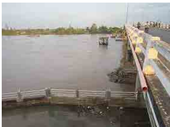
Giao Hoa canal where a sluice gate is needed to prevent saline water from coming into North Ben Tre area
