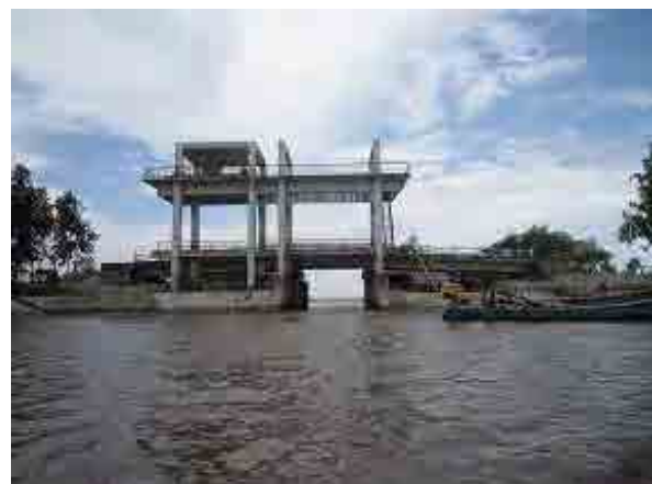
Left photo shows a typical sluice gate constructed in a canal to prevent saline intrusion from coming into inner lands, while the right photo shows a sluice gate constructed at the end point of a canal. The behind of the sluice gate is the West Sea, and this gate prevents sea water intrusion into the canal.
