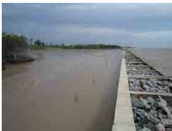
Left photo shows a typical concrete strengthened sea dyke, and the right photo shows mangrove reforestation combined with wave dissipater constructed with concrete frame packed with stones.
