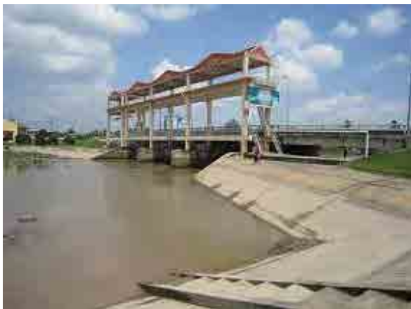
Left photo shows a typical sluice gate constructed in a canal to prevent saline intrusion from coming into inner lands, while the right photo shows a sluice gate constructed at the end point of a canal. The behind of the sluice gate is the West Sea, and this gate prevents sea water intrusion into the canal.
