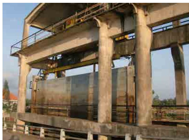
Hoisting device for repairing the swing gate: If the height of swing gate leaf is large, high gate pier is also needed.
