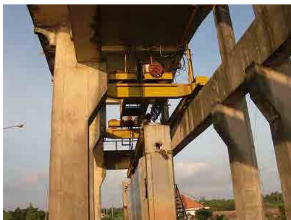
Crane equipped for hoisting and carrying the gate leaf. Crane is usually driven by electric motor.
