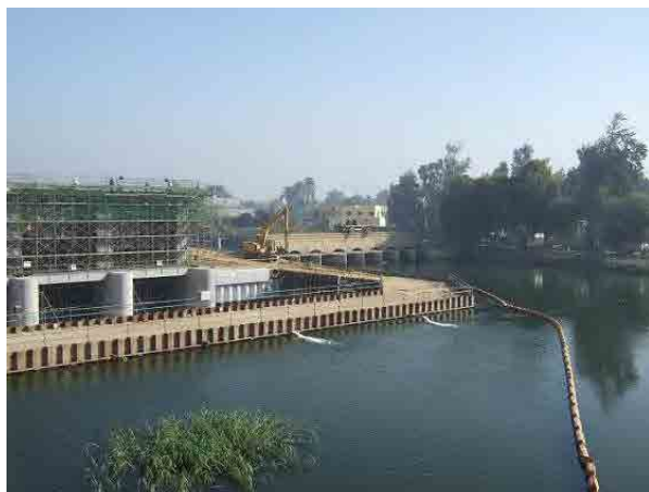
An example of double row steel sheet pile method: Steel sheet pile and filling sand can secure high water-stop ability.
