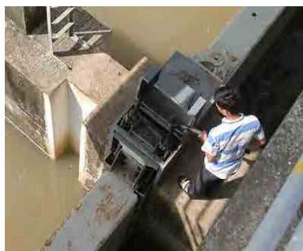
When swing gate is necessary to be closed, operation staff handles the locking device and fixes it.
