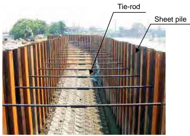
Sectional view of double row sheet piles cofferdam. Sheet piles on both sides are connected with steel tie-rod and the space between the sheet piles are filled by sand
