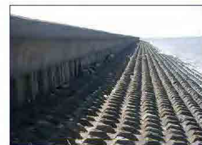
recommended dyke for erosion protection 2.500.000 USD/km
