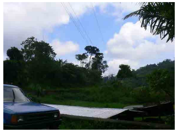
Photograph 8: Existing 13.2 kV power distribution line. Since the existing distribution line (to which the power plant will be connected) uses a lot of wooden poles in poor condition, these will be replaced with steel poles in order to ensure stable supply. Also, 3-phase distribution lines will be used up to the new power plant.
