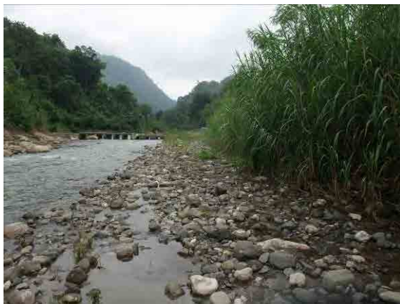
Photograph 7: Current conditions of the power plant construction site. Water will be discharged in this area. There is a road and bridge downstream from here, and it is possible to transport equipment and materials onto the site.
