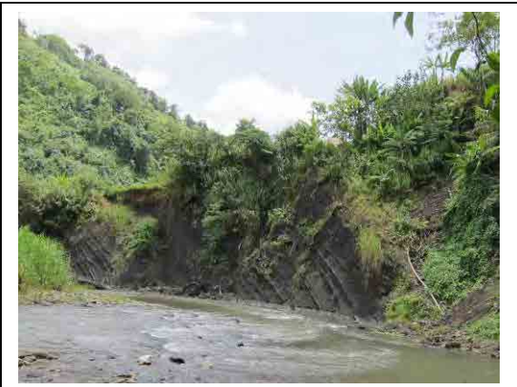
Photo 1-7 (natural condition ; August) undercut slope, where the Lamut river turns left around at TD.500m Central portion of the outcrop is jointed and loosen.
