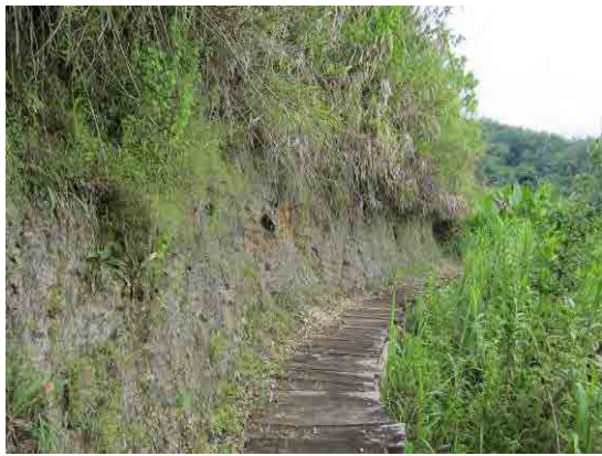
Photo 1-5 Vertically excavated cutting slope on debris to construct the headrace
