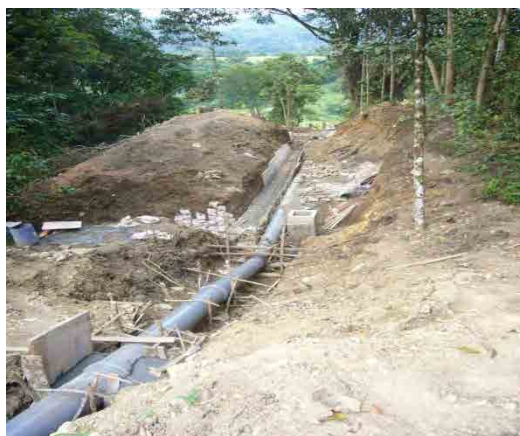
Plate 2-5 Penstock and Spillway 1
