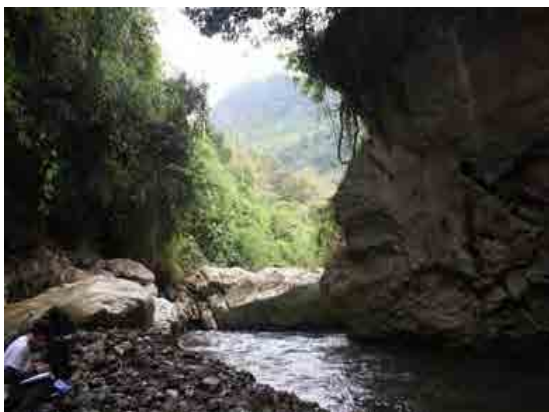
Looking downstream at weir site
