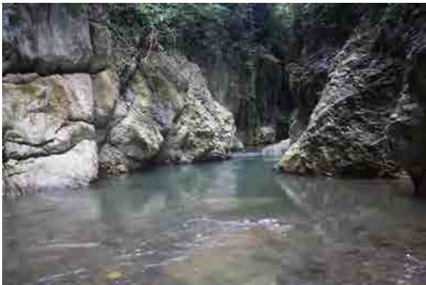
Looking upstream at weir site
