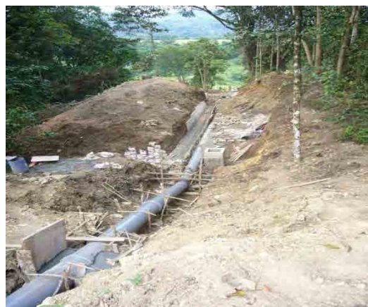
Plate 2-5 Penstock and Spillway 1
