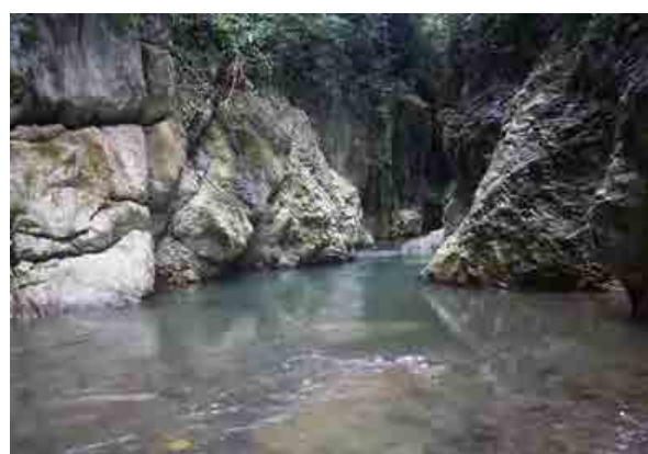
Looking upstream at weir site
