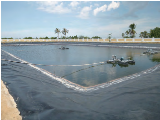
Figure 4.7.13 Domestic Water treatment Plant in Phan Rang (first pond)
