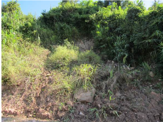
Photo 1-15 Collapse on the Upper Slope of the Powerhouse, which Occurred in a Highly Water- contained Loosen Cohesive Soil
