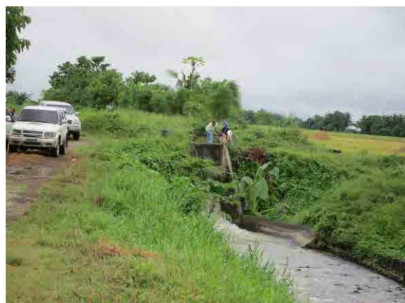
An embankment is exposed, and collapse is seen here and there to lower the waterway in the harvest time. However, the concrete structure of the weir is not damaged.
