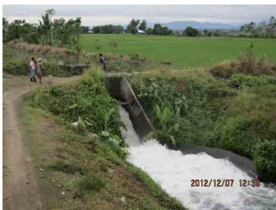
Photo-3: Approximately 3m-high water head at downstream of the existing drop work is currently untapped. On both sides of the drop work, the Project will install simple turbines.
