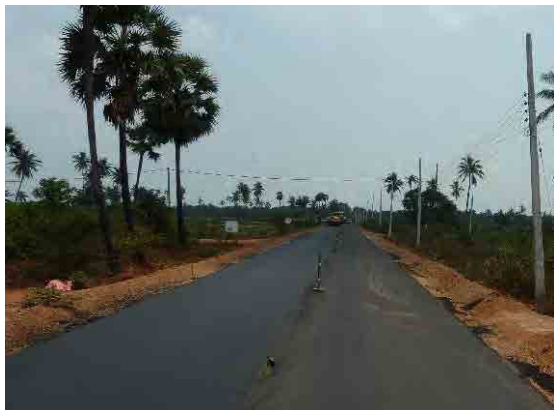
Picture 2e: Rehabilitation of Road
