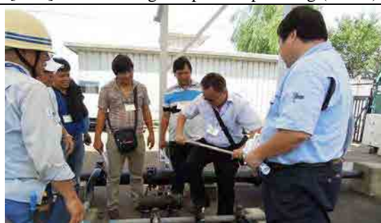
[D08] Service pipe installation training (Jul.27)
