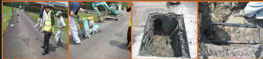
It was measurement of trace amount of water from PVC pipe leak from a needle hole
