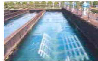
Cross Flow Paddle type Flocculator
