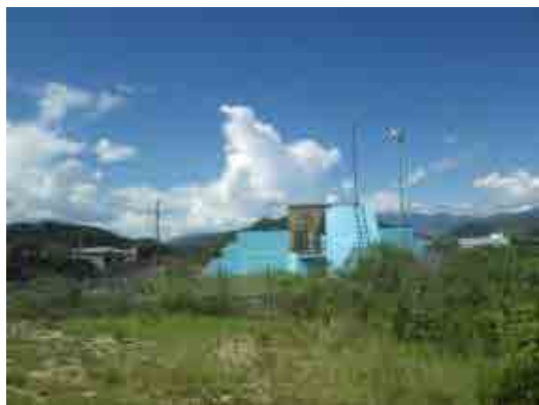
Photo 1-3-1 Planned Powerhouse Construction Site in Concepcion Site
