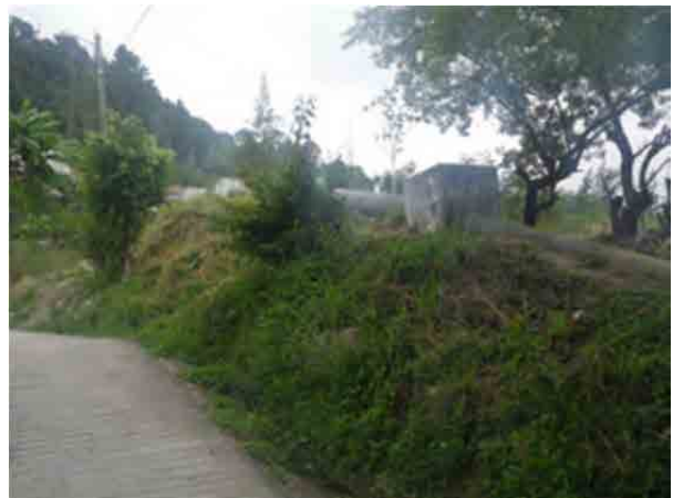
Photo 1-3-6 Existing L22 pipeline at Picacho Site
