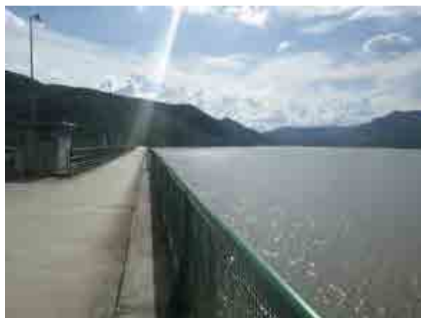
Photo 1-3-4 Reservoir of Concepcion Dam
