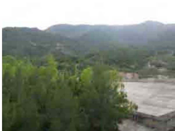
Photo 1-3-3 Upstream of Concepcion Dam
