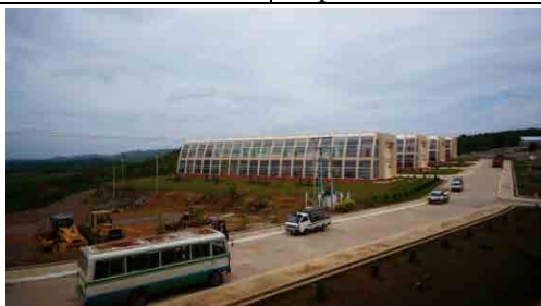
Still building new facilities
