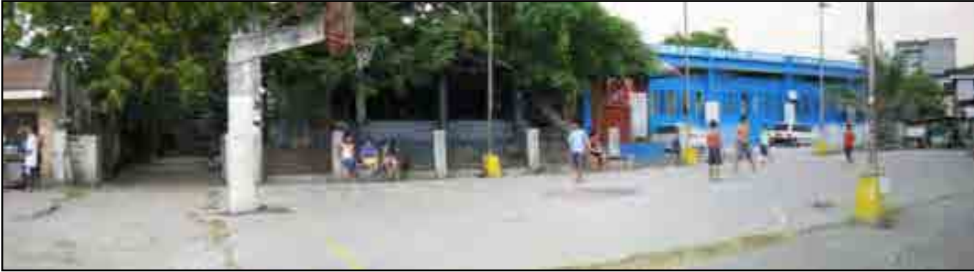
FIGURE 7.4.4-2 ABANDONED FORMER BUREAU OF LAND TRANSPORTATION BUILDING WHICH IS NOW USED AS THE PNP AVIATION SECURITY GROUP K-9 OFFICE. THE COMPOUND CAN SERVE AS A RELOCATION SITE FOR THE INFORMAL SETTLER PAPS WHOSE COLONY IS ADJACENT TO THE STRUCTURE
