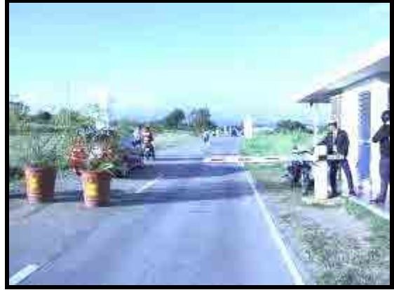
Plate No. 6 Photo taken along the Nuvali Road. The properties on both sides of the road are owned by the Greenfields.
