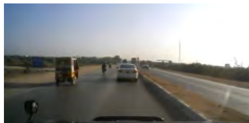
Photo 5.4-2 Road in Karachi District
