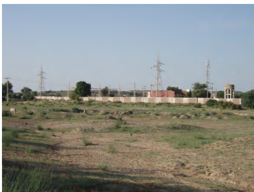
Photo 5.1-1 66 kV Islamkot Substation
