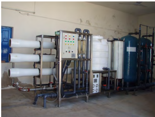
Photo 5.2-1 Existing RO Plant (#4)
