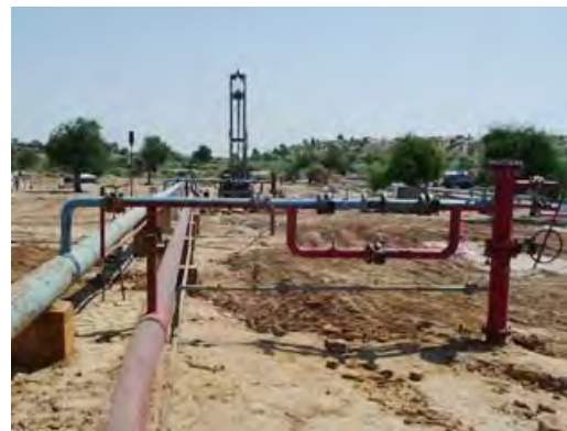
Photo 4.3-2 Air and Gas Pipelines
