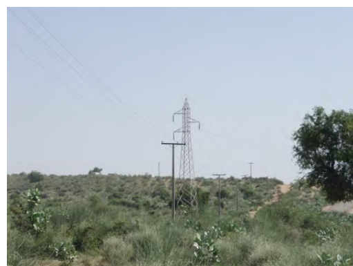
Photo 5.1-2 66 kV Transmission Line
