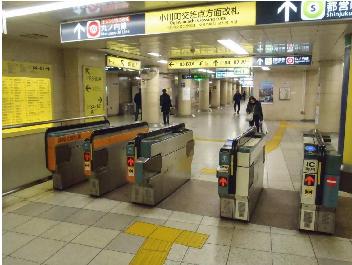
Figure 9.2 Example of gates of Automatic Fare Collection system (AFC)
