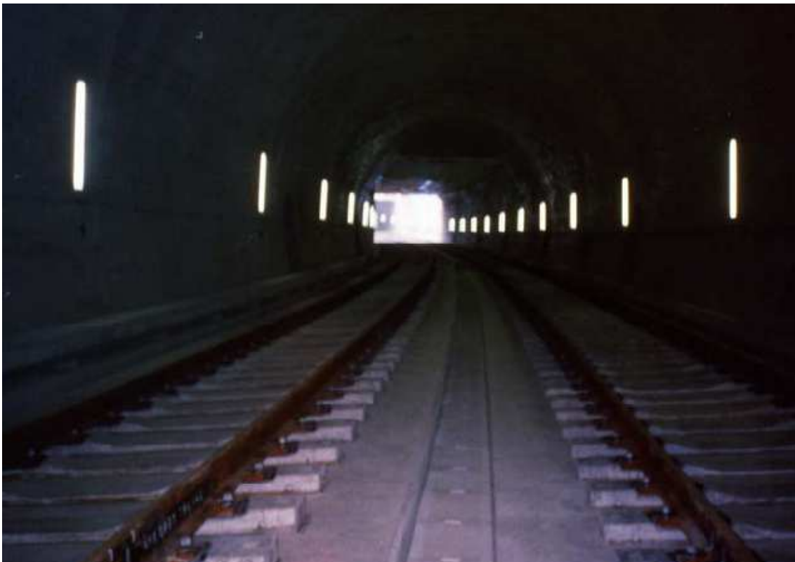
Example of railroad ties anti-vibration system
