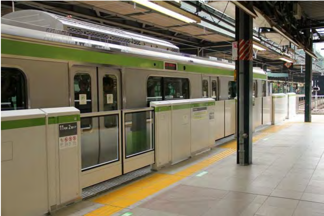
Example of half size Platform Screen Doors (PSD)
