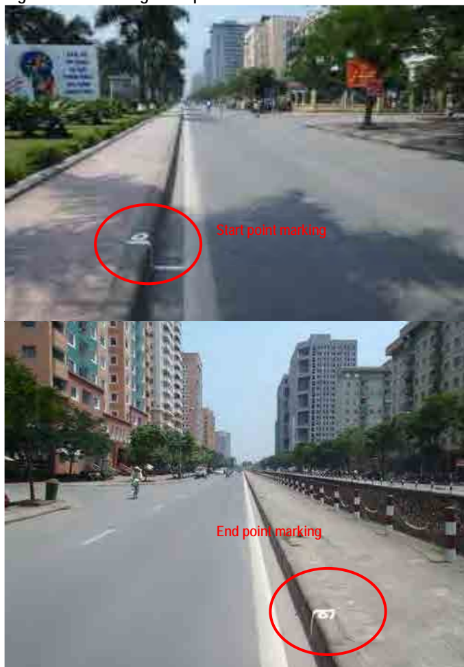
Figure 2.15 Marking Example – 1 km Distance
