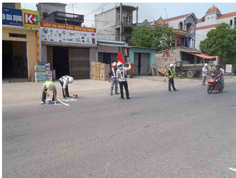
Figure 51 Safety Keepers Working During Marking (Field Reconnaissance)
