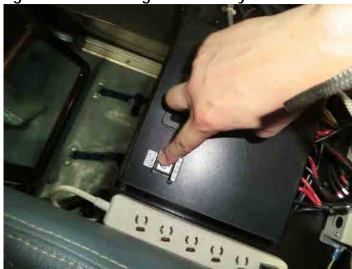
Figure 3.30 Shutting Down the System
