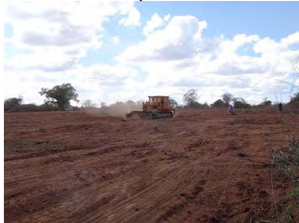
Site preparation Kibwezi
