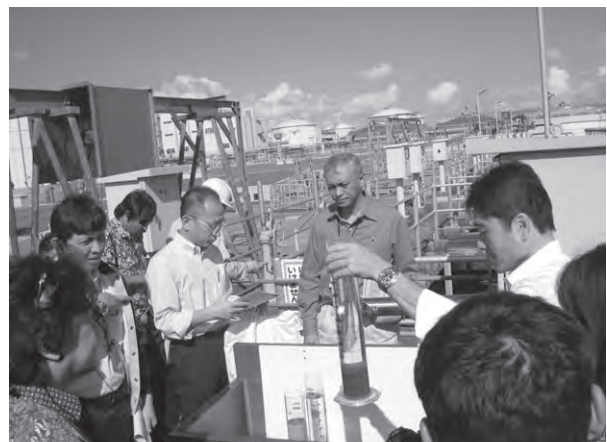
2/10 Hiagari Wastewater Treatment Plant
