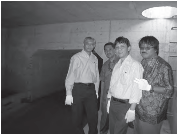
1/10 Storm Overflow Chamber at Kimachi Park
