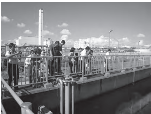
2/10 Hiagari Wastewater Treatment Plant
