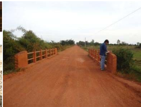
Photo 12-4 Concrete bridge(1 lane)
