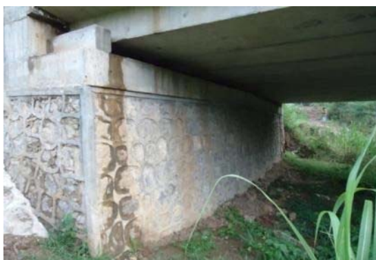
Photo 3-9 Masonry abutment
