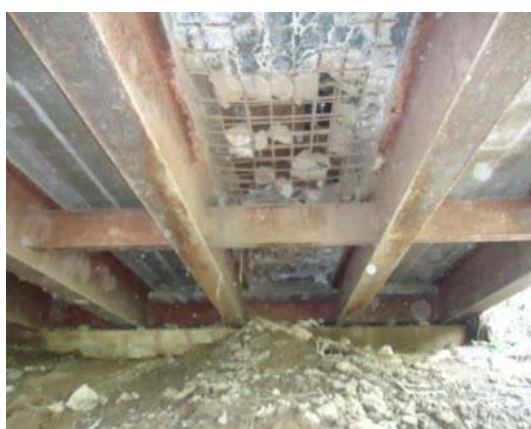
Photo 3-17 Bridge on NR21
