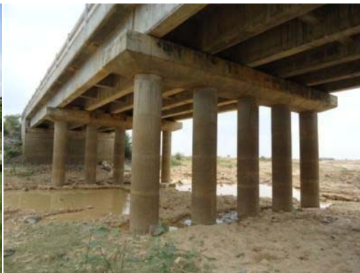
Photo 3-6 Concrete Bridge (T girder)
