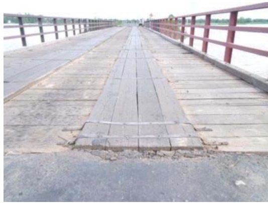
Photo 3-4 Wooden deck on steel bridge
