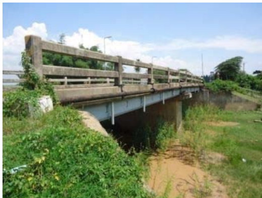
Photo 3-5 Steel Bridge (I girder)
