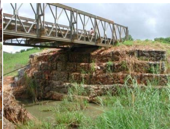
Photo 3-8 Gabion abutment
