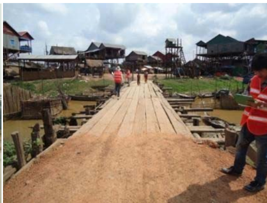
Photo 3-20 Bridge on PR265C
