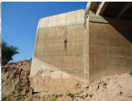
Photo 3-18 Bridge on NR64
