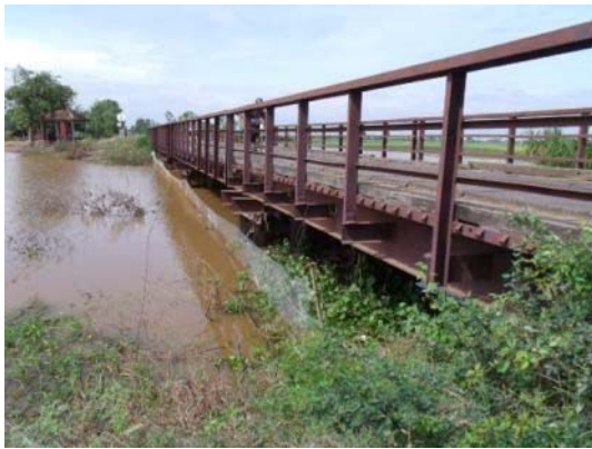
Photo 3-3 Steel bridge (Temporary type)
