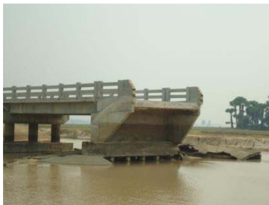
Photo 3-19 Bridge on PR312B
