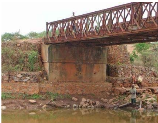
Photo 3-7 Concrete abutment
