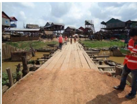
Photo 3-4 Bridge on PR265C
