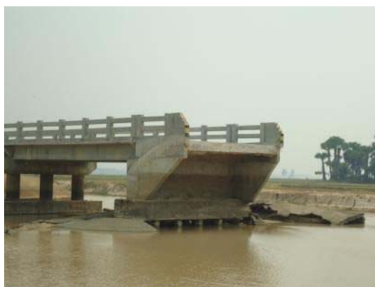
Photo 3-3 Bridge on PR312B
