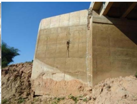
Photo 3-2 Bridge on NR64
