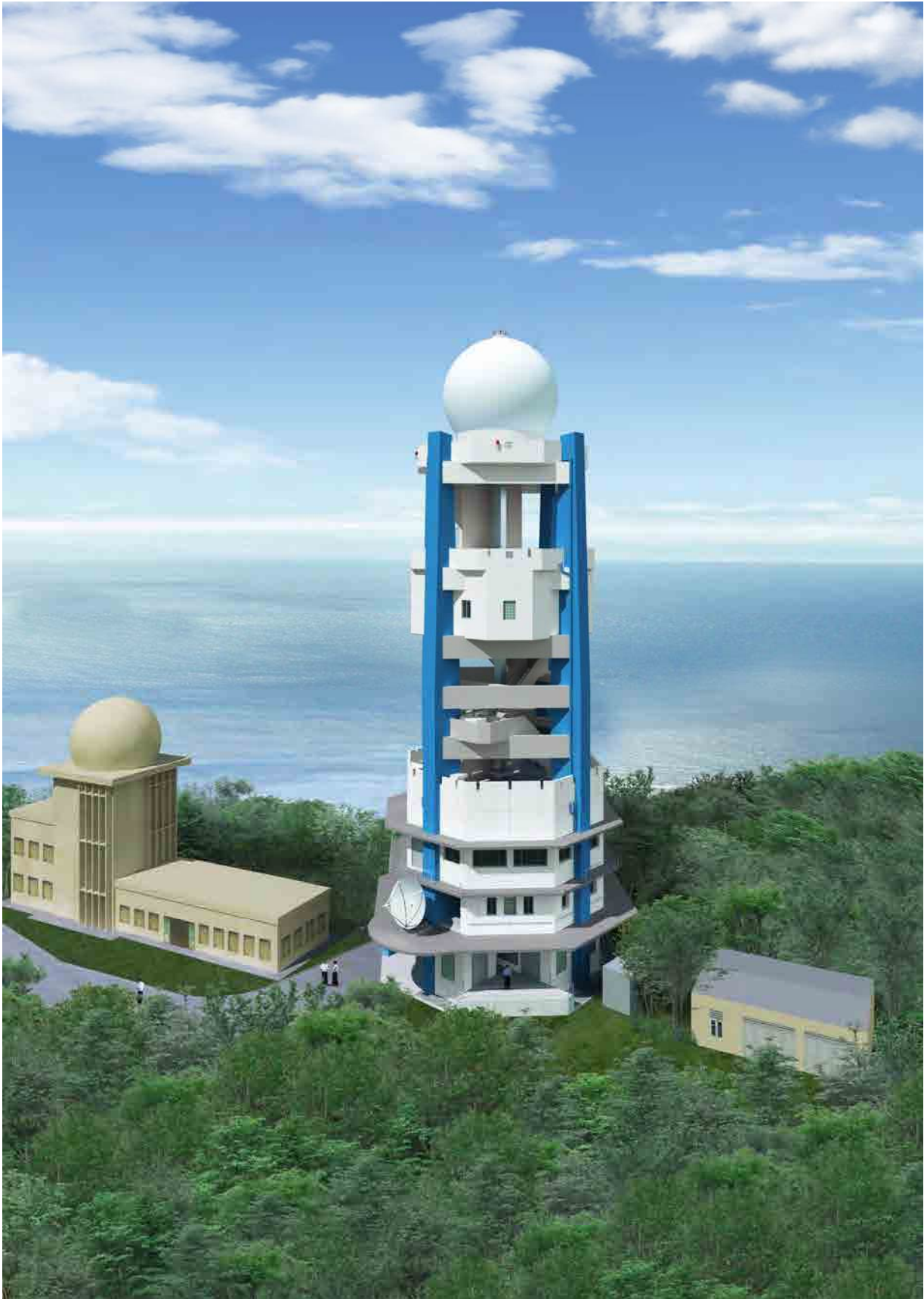
Kyauk Phyu Meteorological Radar Tower Building
