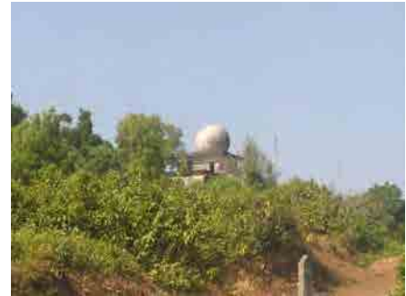
Kyauk Phyu Meteorological Radar Observation Station
