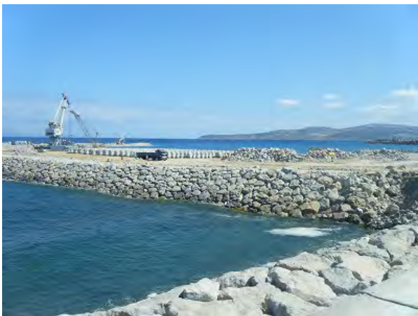
Fishing Port, under Construction,
